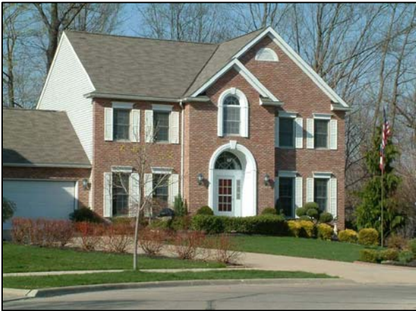
New construction of a larger single-family home
