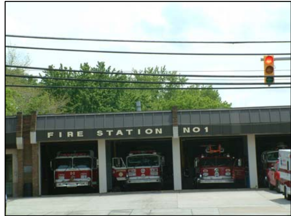
Brooklyn Fire Station - existing
